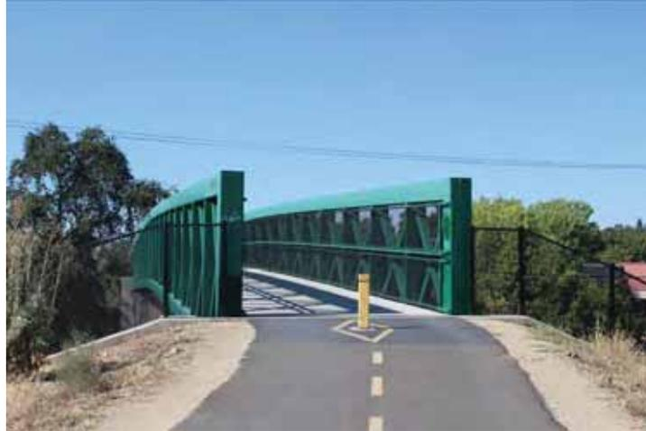
**Figure 5 -- Prefabricated Truss Bridge**
